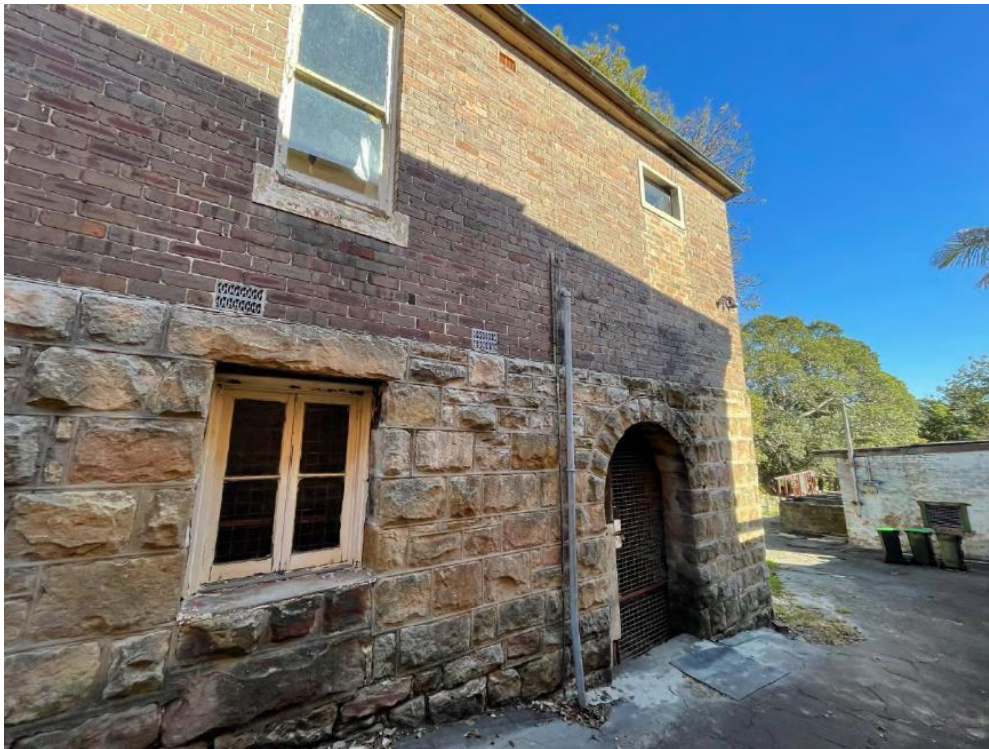
Figure 12: Existing sandstone base, proposed to be used as lower ground level art studio that can also function as a separate, self-contained dwelling – new timber framed stained glass window proposed to arch
