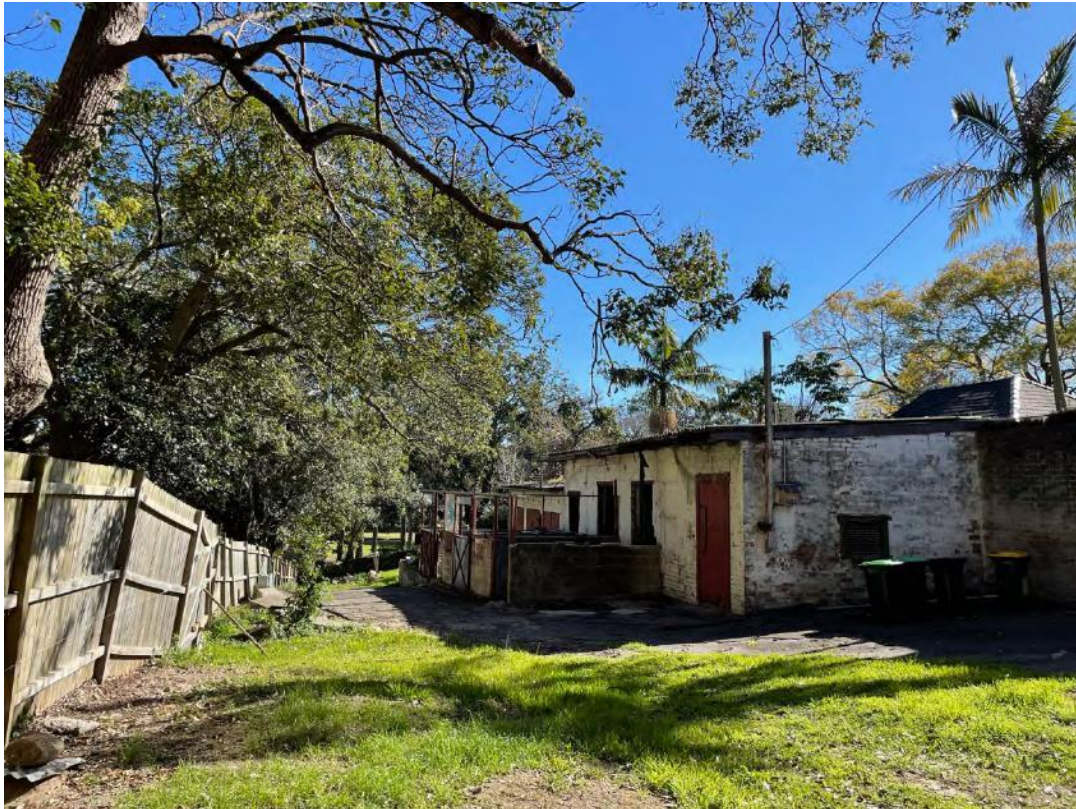
Figure 15: Looking north-west on site, stable block to right of image to be demolished
