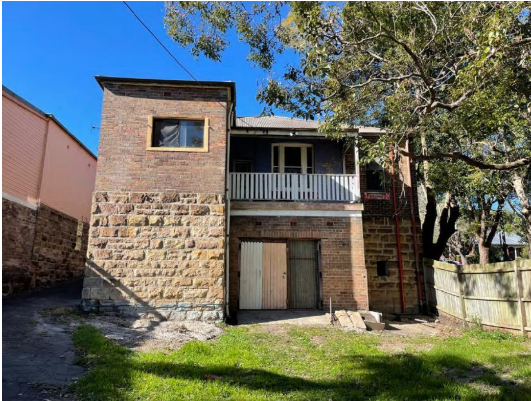
Figure 13: Rear of existing dwelling on site
