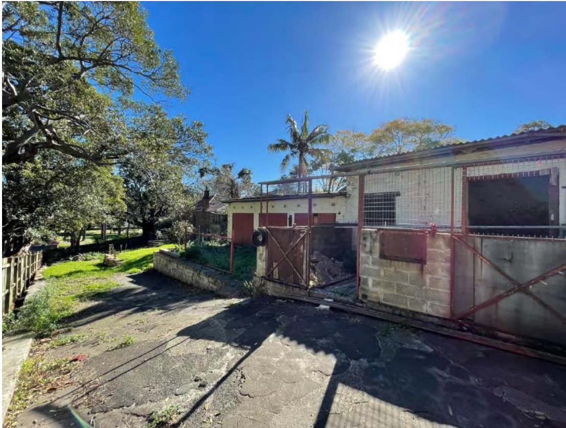
Figure 17: Stable block and rear of site, looking north toward 1 Alexandra Lane
