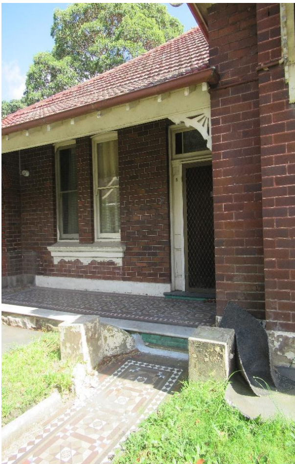
Figure 46: Masonry plinths to be removed
