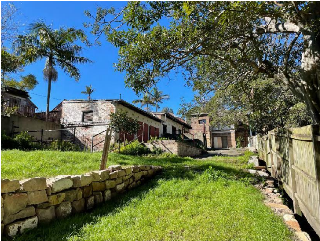
Figure 19: Rear of stable block and existing dwelling as viewed from backyard, looking south-east
