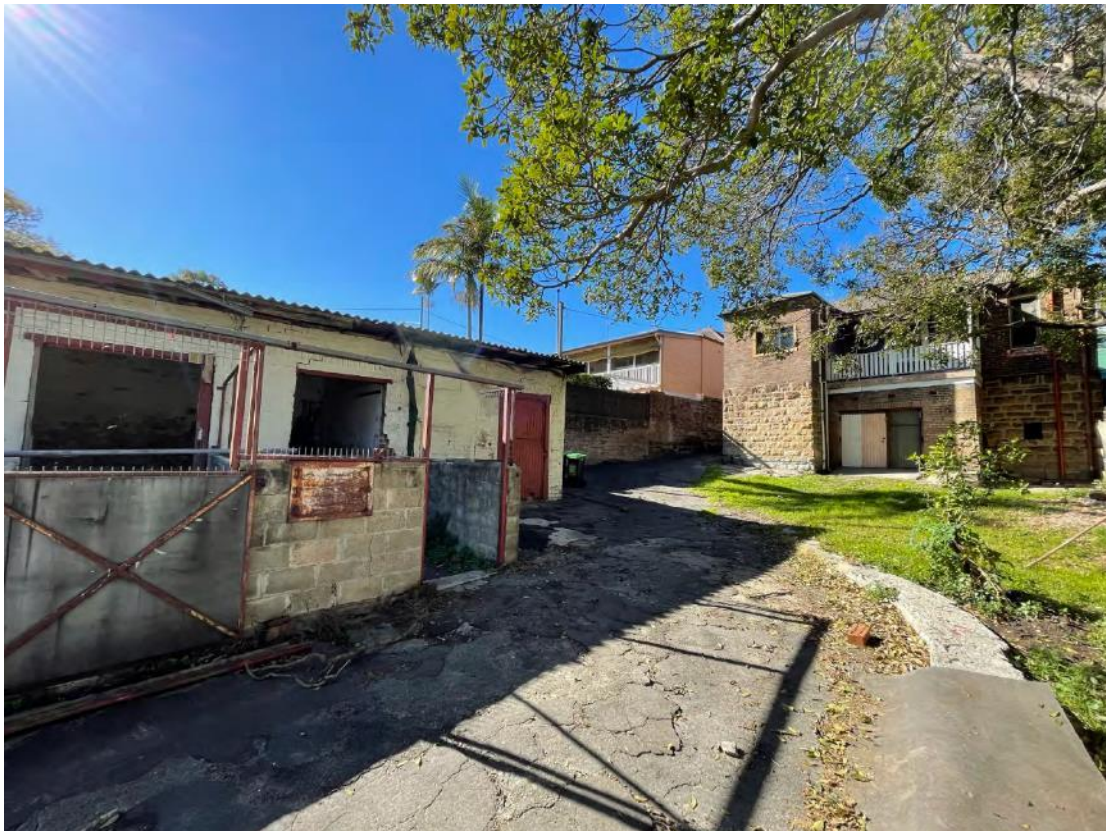
Figure 16: Stable block and existing dwelling, looking east on site
